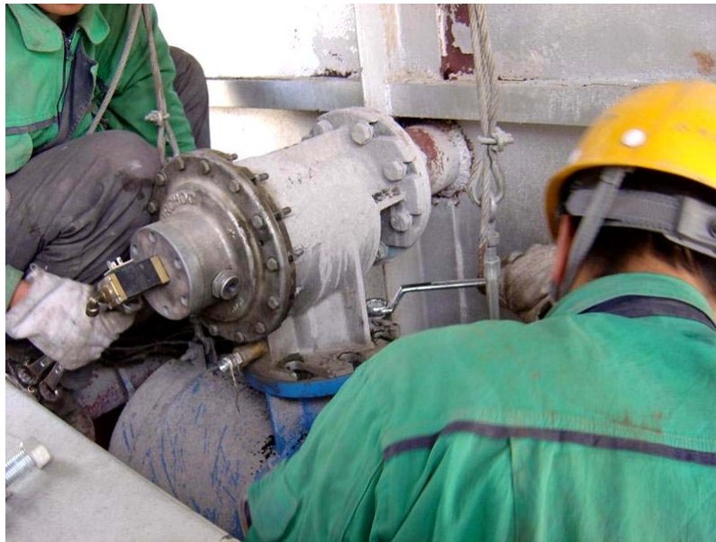
Existing blasting head removal
